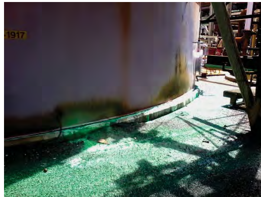
Figure 6: A bright green deposit was found around the perimeter of 360-1917
