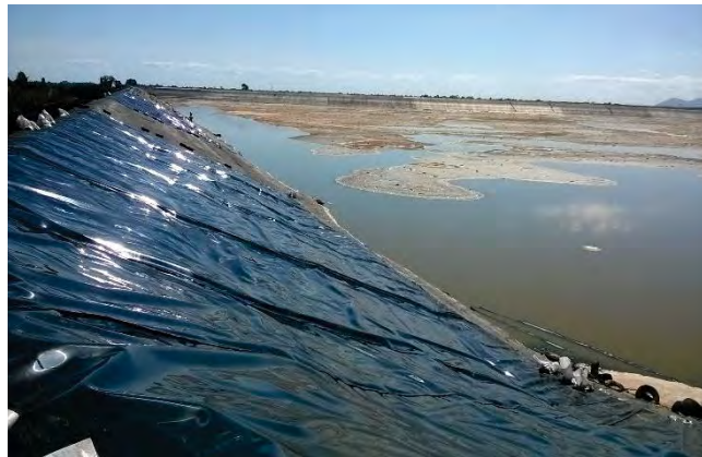
Figure 8.9: Repairs to Brine Dam
