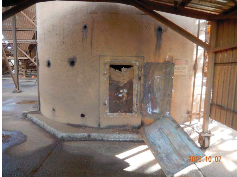
Figure 7: Accumulation of debris at base of stack
