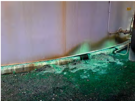
Figure 5: Damp spots found on the concrete berm of 360-1917
