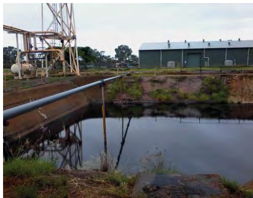
Photo of the oil dumped in the newly extended bund- AHS sphere
