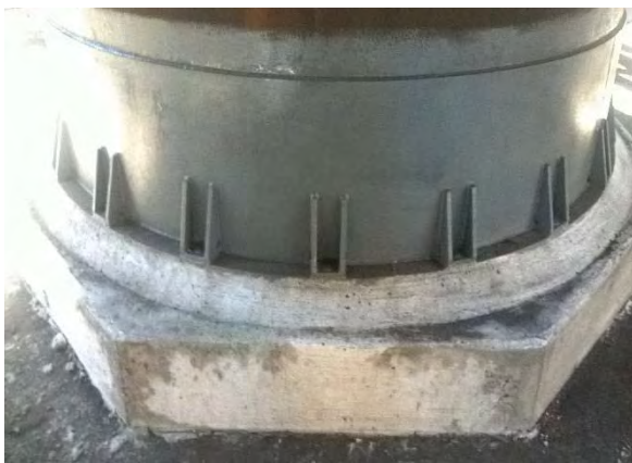
Figure 8.5: Example of repairs made to 352 Tailing Stills
