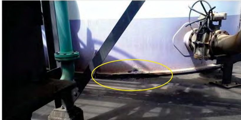
Figure 4: Significant signs of corrosion sighted in the floorplate of 355-1961
