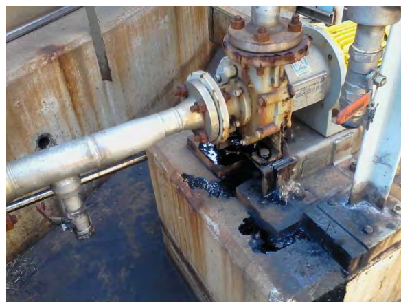
Figure 8.13: Leaking organic solvent from pump connected to 356-19201
