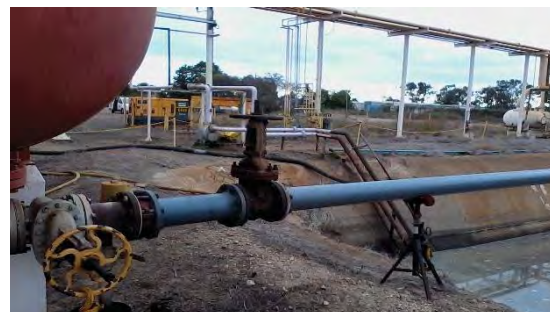
Figure 8.2: Installation of automated dump valve on 450-1909 Oil Tank
