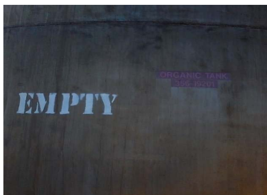
Figure 8.10: Incorrect marking on 356-19201
