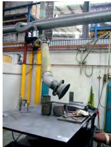
Welding fumes are extracted via flexible, locatable forced extraction and ventilation system.
